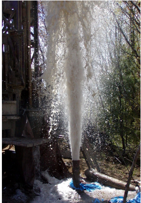
Installation of an HSA-sited test well
