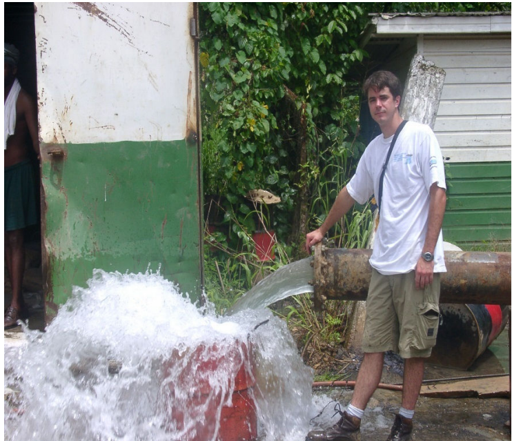
HSA Project Manager Supervises Pumping Test of 1,100 gpm Well
