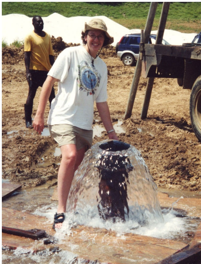
HSA-sited and developed well exhibiting >450 gpm of natural artesian flow that has now continued unabated for over 15 years.
