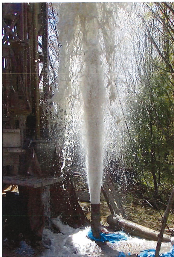
Installation of an HSA-sited test well
