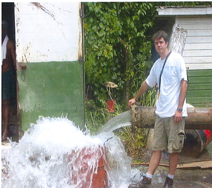
HSA Project Manager Supervises Pumping Test of 1,100 gpm Well
